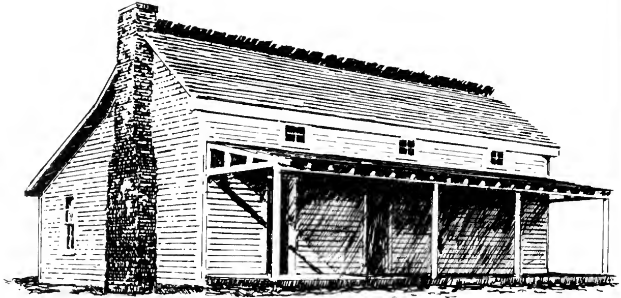
LOG HOUSE WITH CLAPBOARD SIDING
